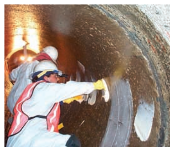
Tyfo® WP (Wet prime) & TC (Tack Coat) epoxy prime coats to enhance bond strength
