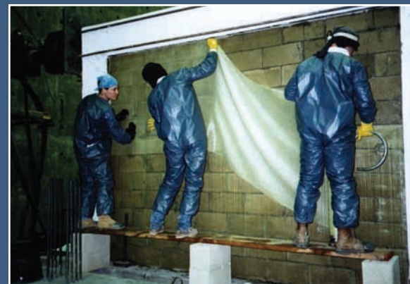
Seismic strengthening of masonry-infilled frames using the Tyfo® SEH System
