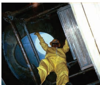
All required materials and labor are inserted through existing manholes
